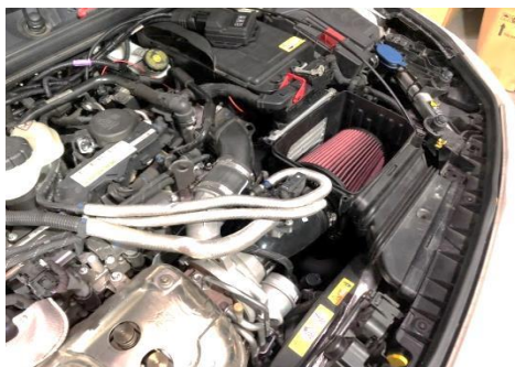
Figure 29: Prepare to install the MST heat shield "A"
